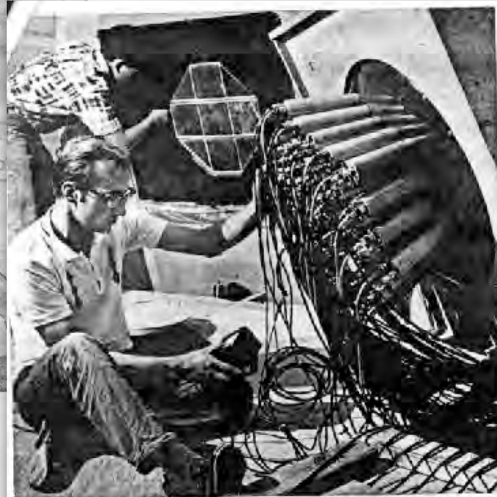
Graduate students at work in the "Cosmic House," their nickname for the unusual observatory. At left, Alan Zabel, Brooklyn, New York, mounts a filter over an observing aperture, while Fred Ruckdeschel, Whitestone, New York, checks out a bank of phototube preamplifier bases. At right, Mr. Zabel and Roscoe E. Marrs, Schenectady, New York, mount cathode-ray tubes in the camera-room display.
