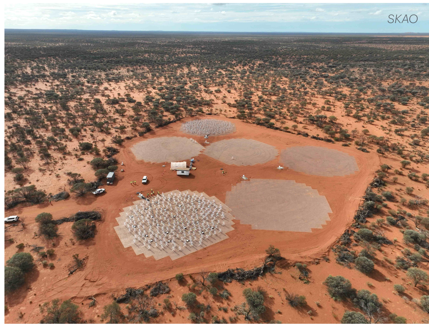
The first 2 complete stations with 512 antennas, deployed at Murchison Radio-astronomy Observatory
