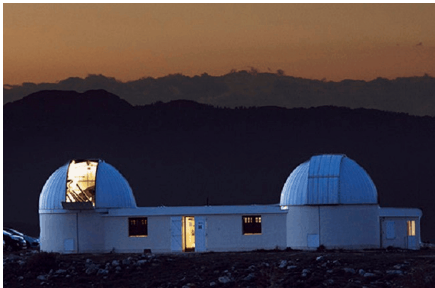
C2PU Calern (France)
