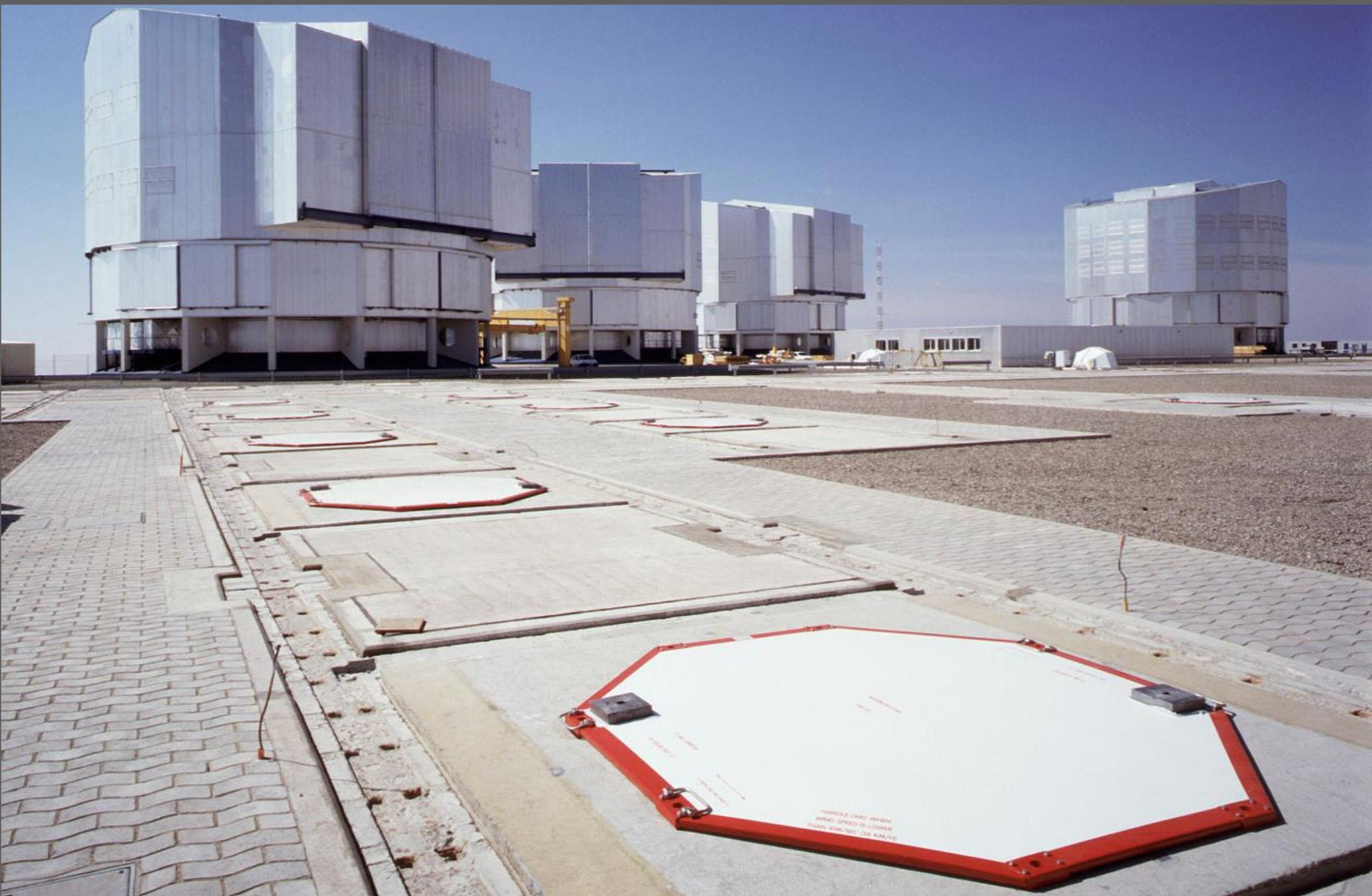
VLTI stations for auxiliary telescopes, above the ducts that lead to the interferometric tunnel
