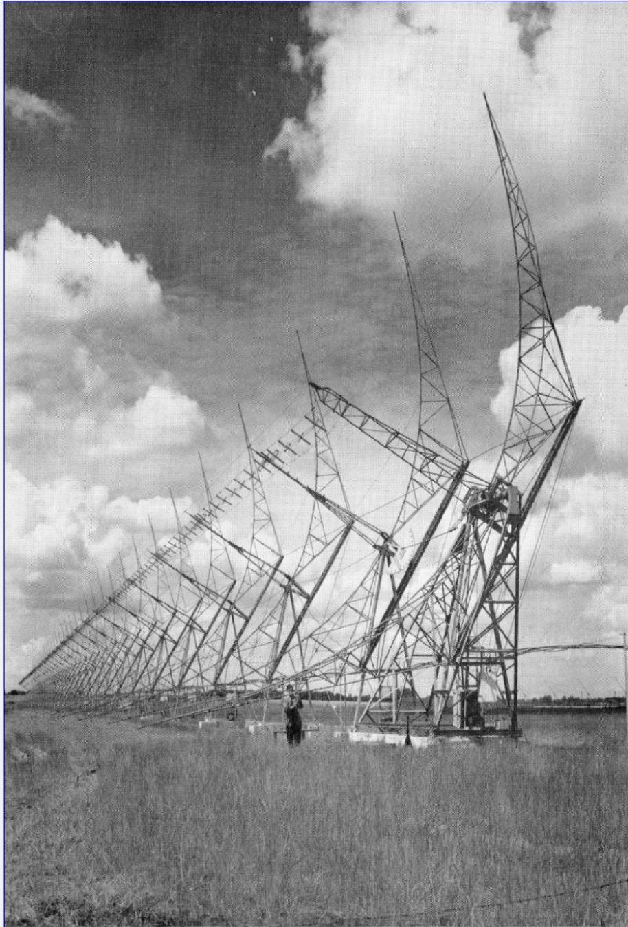
*The long fixed element of the radio star interferometer.*
